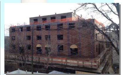
Brick Work in progress
