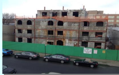
4 th Floor Work Completed
