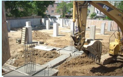
Foundation Work Completed
